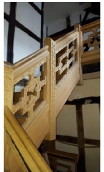
Figure 7: Image of the reconstructed staircase at the Staircase House in Stockport
